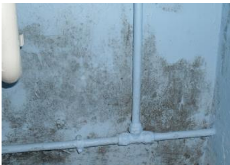
FIGURE 3: The dampness and mould in many kitchens, bedrooms and bathrooms is a major cause of health issues among residents
