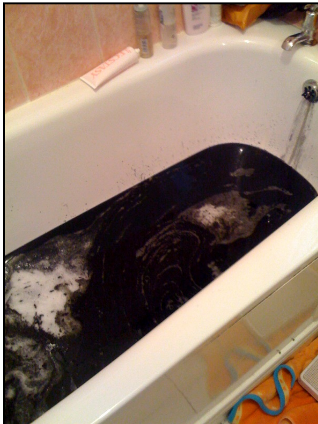
Plate 2-3 Wastewater Backup Observed on June 28 th 2010
