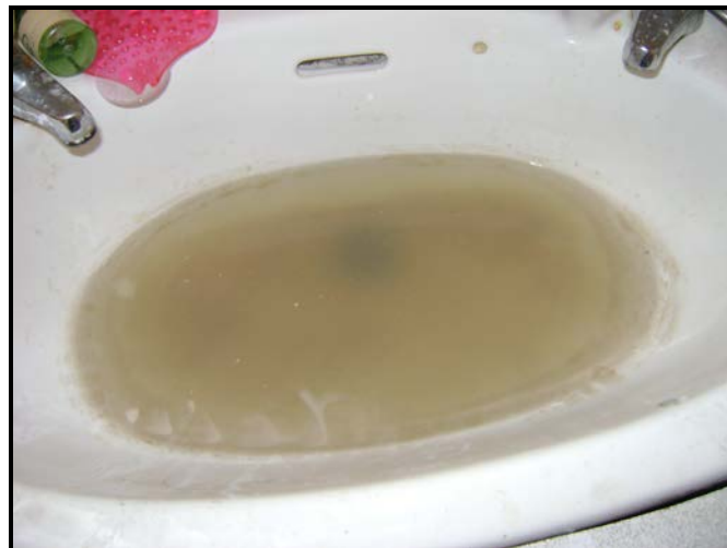
Plate 2-1 Wastewater Backup Observed on 13th May 2010 – House No 144
